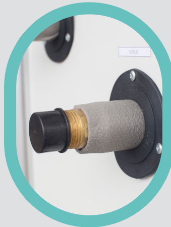
Extended stubs and additional insulation
